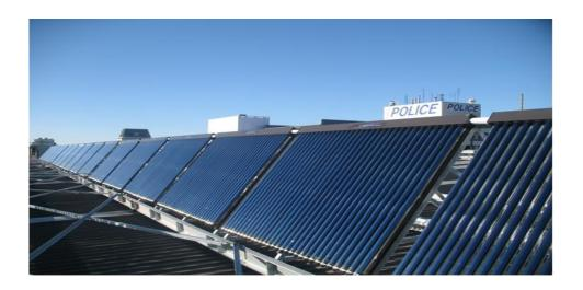
Consol 30-58-1800 Collector Flat mount on Corrugate roof Valve vent, Open loop
