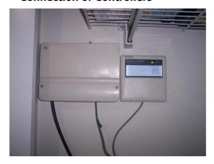
Installation and commissioning of the controller must be carried out by a registered electrician and in accordance with the operation and instruction manual. Care should be taken when wiring in the controller auxiliary heating where ripple control could disturb the operation of the system. The adjustment of controllers may adversely affect solar performance.
